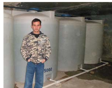
Ramani, a Dzegvi resident, who helped build the new water system
